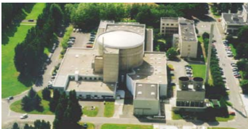
Fig. 1 : View of the Orphée reactor, guide hall and laboratory buildings.
